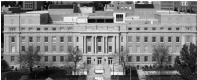
Chamberlin Hall viewed from the new Chemistry Building addition.
