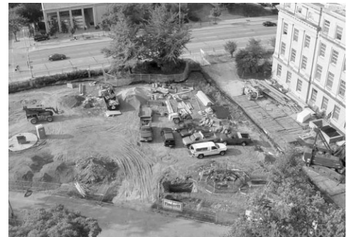
Newton Apple Tree at the beginning of new Botany Garden construction.
